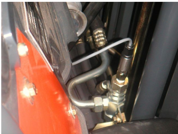
Typical Hydraulic Pressure Transducer Installation
